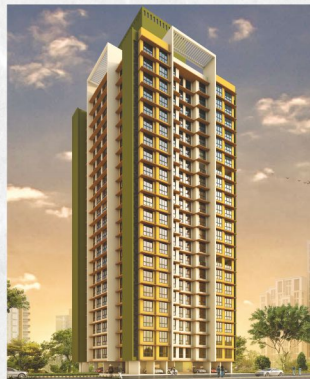
ADITYARAJ AVENUE VIKHROLI
