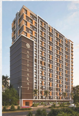
ADITYARAJ SPRINGS CHEMBUR
