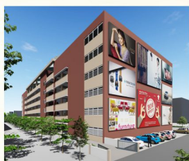
PARKING TOWER BUILDING CBD BELAPUR
