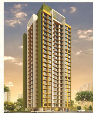
ADITYARAJ AVENUE VIKHROLI
