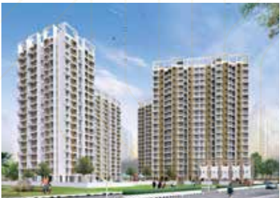
NAKSHATRA GREENS PH. 1 & 2 Naigaon (East) Phase I MahaRera Regl. No.- P99000005051 Phase II MahaRera Regl. No.- P99000008753
